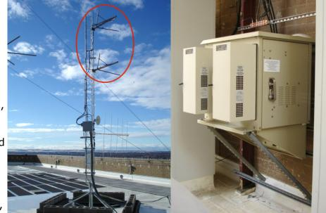
Two-bay low power antenna attached to a rooftop tower
