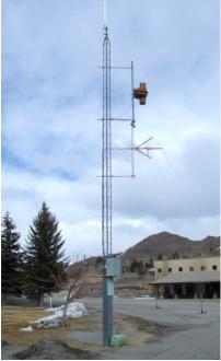
Tower with two co-located low power antennas connected to transmitters in building closet via 140ft underground conduit
